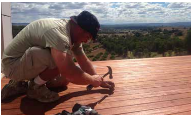
Troy putting on the decking boards for the central deck areas.
